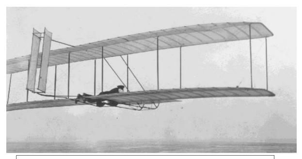
While readying their powered Flyer 1, the Wrights modified the tail of the 1902 glider, adding a second movable vane to give the rudder more authority.
